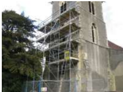
Scaffolding around the tower for rendering repairs - Photo: Tony Hughes
