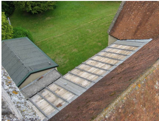
Photo: The north aisle roof stripped of lead, July 2019; Tony Hughes
